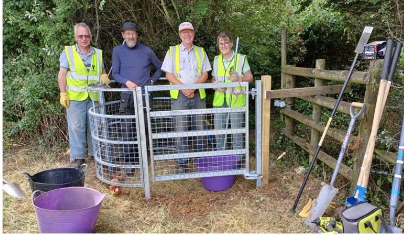
Bob Merry, second from right, with other members of Thame and Wheatley group's path maintenance team, having just installed a kissing gate in Holton parish. Photo by a passerby.
