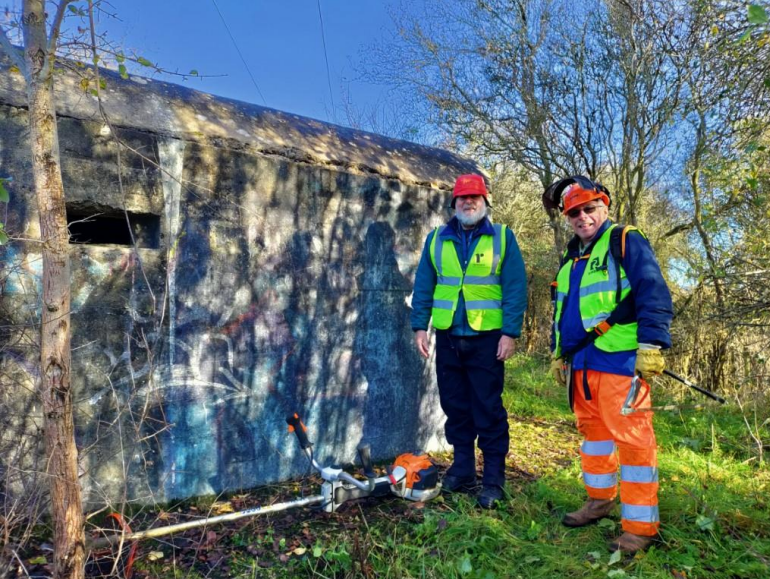
John and Pat alongside a pillbox on the western edge of Abingdon. Photo Dave Cavanagh.
